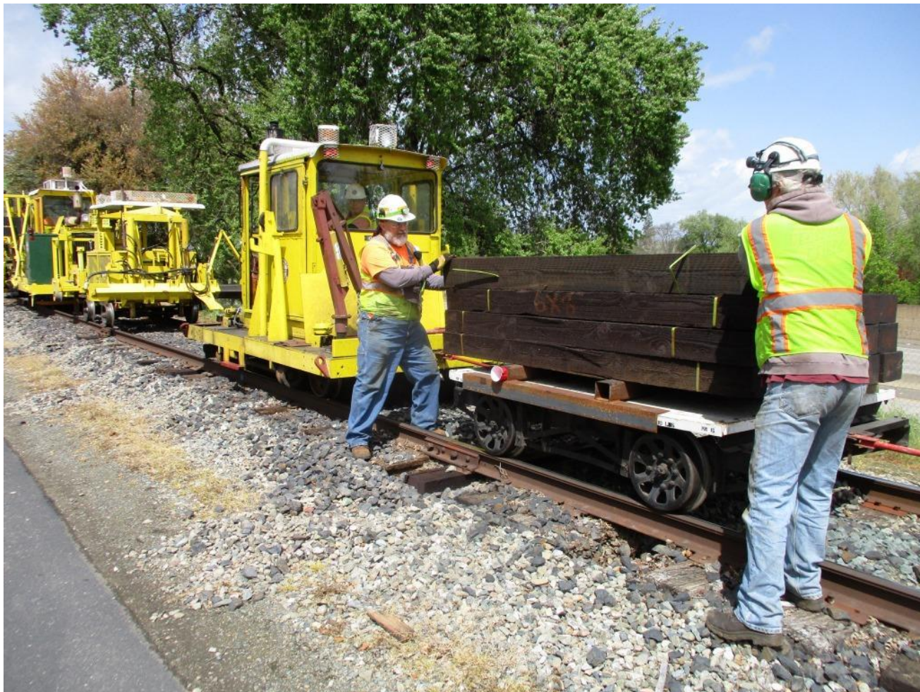
With Bill at the throttle of the Kalamazoo, Mike F. and Steve deploy new ties for insertion
