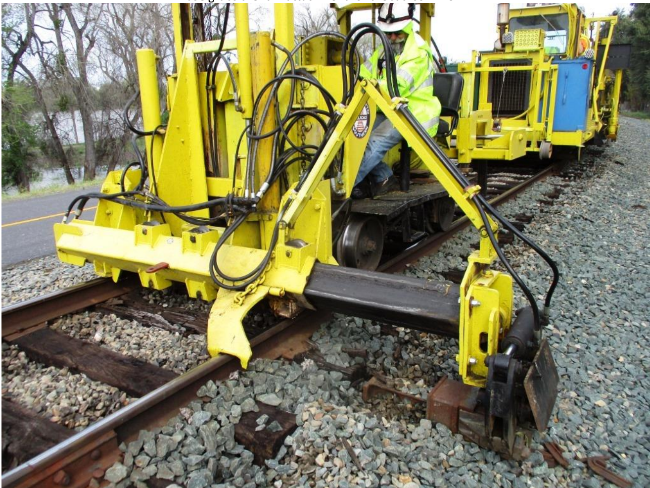
...And uses it to shove out a tie that shattered when an attempt was made to pull it
