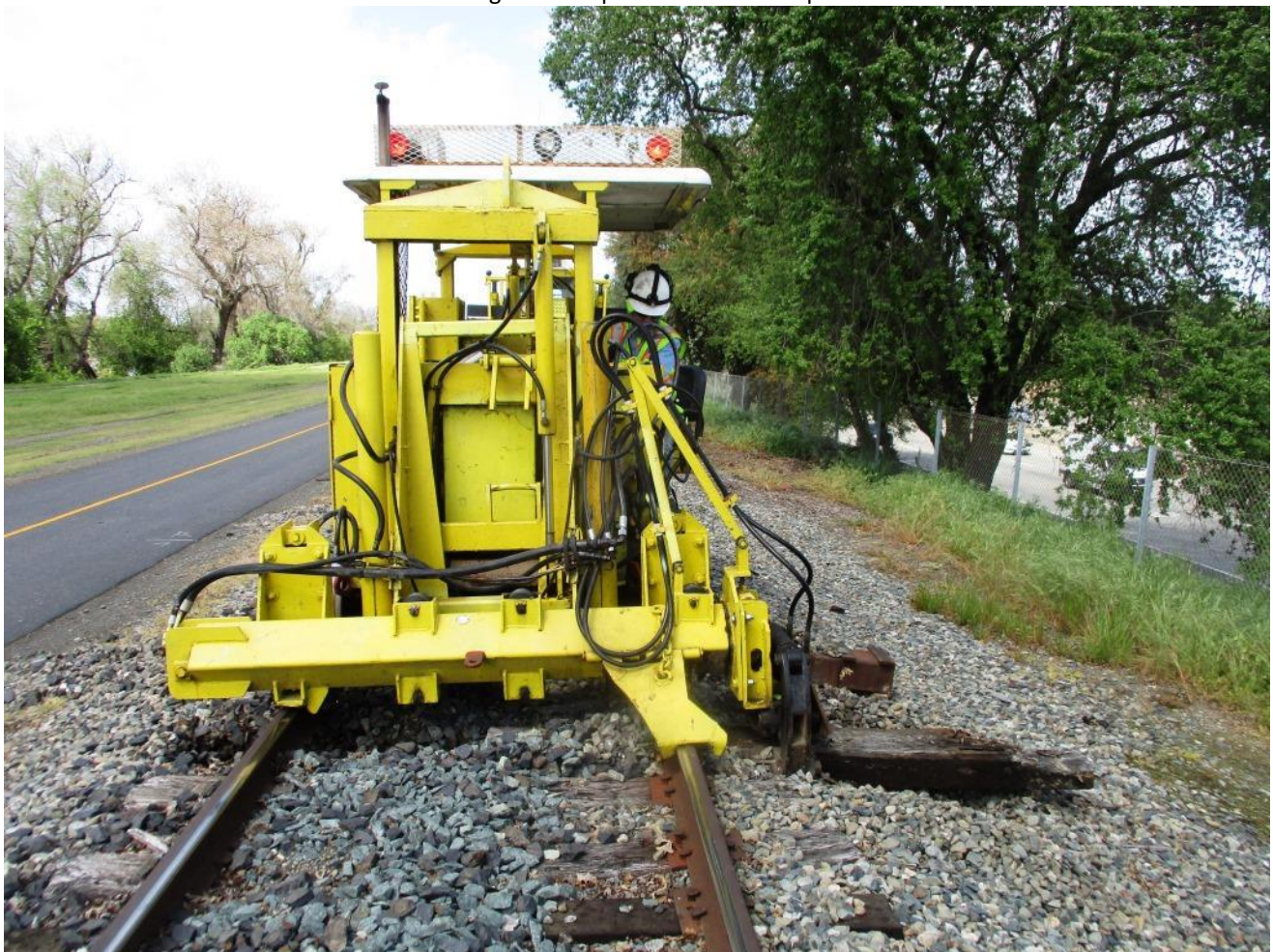
Joe carefully pulls a busted tie with the Jackson 125
