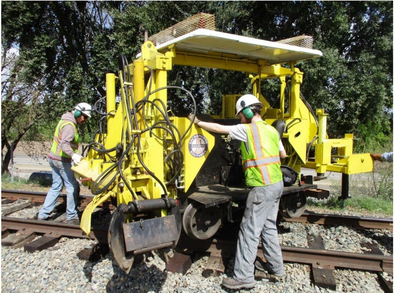
Matt and Steve spin the Jackson 125 around to grab the shoved ties from the west side of the track
